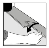
**2.** To engage the locking system, press the end of the board until you hear a click. A click indicates that the locking system is properly engaged.
